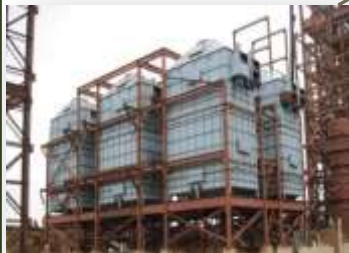
COAL GASIFICATION PLANT FOR JINDAL STEEL
