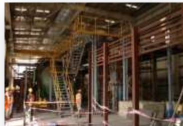
COLOUR COATING LINE FOR TATA BLUESCOPE LTD.
