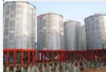
SILOS AT KFL, KERALA
