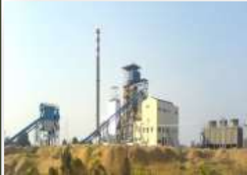
10 MW POWER PLANT FOR VARUN BIO ENERGY
