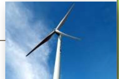
1.5 MW WIND TURBINE AT UTHUMALAI
