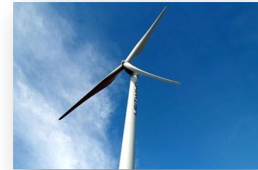
1.5 MW WIND TURBINE AT UTHUMALAI
