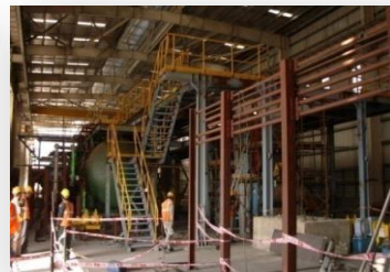
COLOUR COATING LINE FOR TATA BLUESCOPE LTD.
