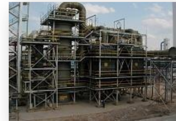
GAS CLEANING PLANT FOR KCM, ZAMBIA
