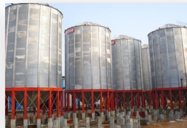
SILOS AT KFL, KERALA
