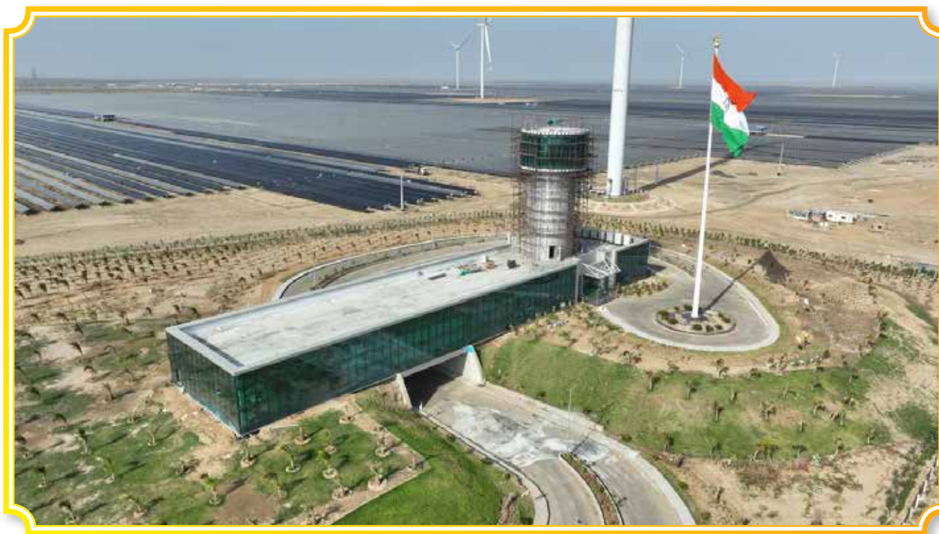
Khavda Renewable Energy Park, Gujarat financed by REC
