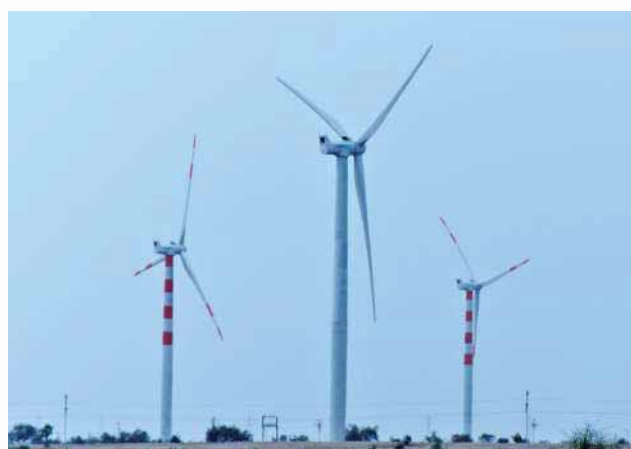
OIL has considerable presence in Low Carbon business like Renewables. View of a Wind energy Generation site in Rajasthan
