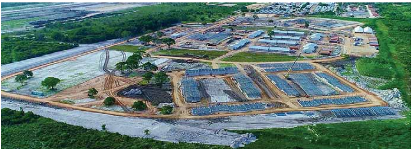
Aerial view of Camp Expansion activities at Mozambique
