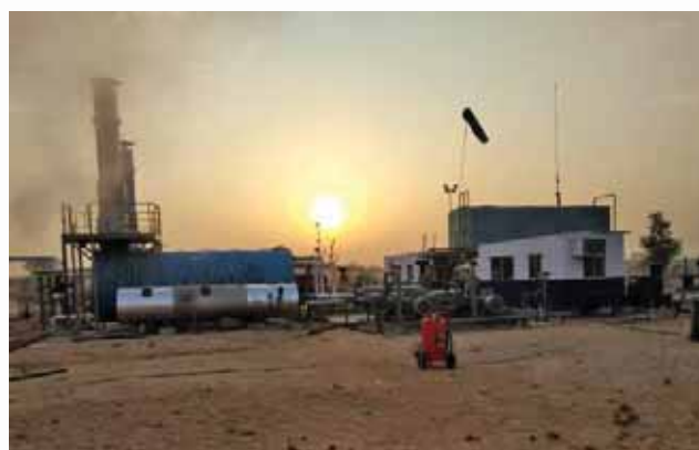
A natural gas production Installation at Baghewala, Jaisalmer, Rajasthan
