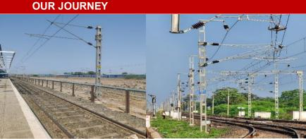
Balance Work of Electrification of 3rd line between Vilayatkalan Road (VYK) to New Katni Junction (NKJ) including modification of yards by 2x25KV, 50HZ A.C, single Phase Over Head Equipment In connection with Anuppur- Katni 3rd Line in BSP Division Over S.E.C. Railway.
