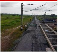
Electrification of doubling line including Cross overs between Urkura to Raipur store depot. (approx. 2.150 RKM/3.5TKM) by 2 x 25 KV AC OHE system in Raipur division over S.E.C Railway
