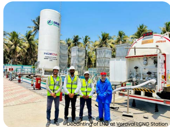
Decanting of LNG at Veraval LCNG Station
