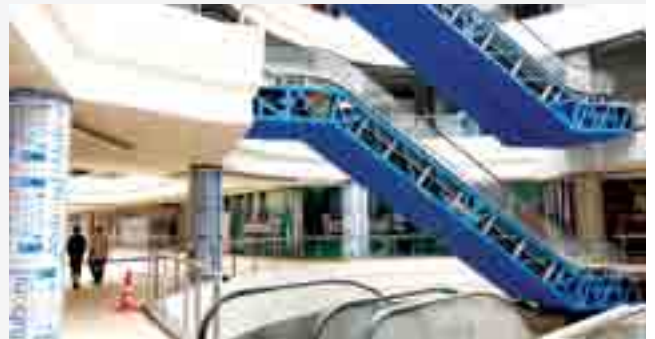
Fitouts and MEP in progress
