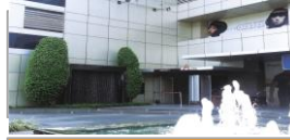
Phoenix House, Mumbai
