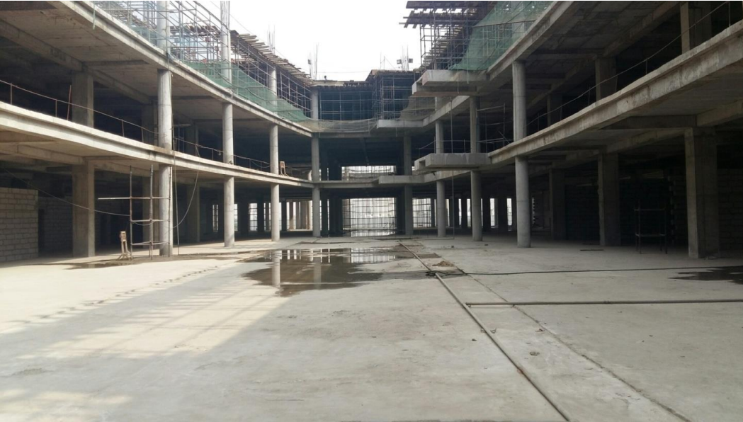
Upper Ground Atrium
