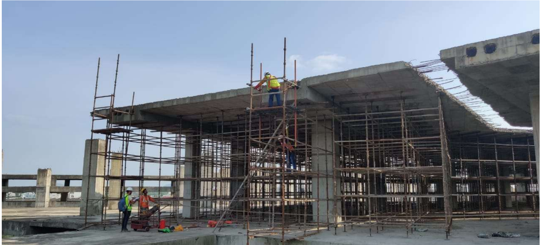
Construction in Progress
