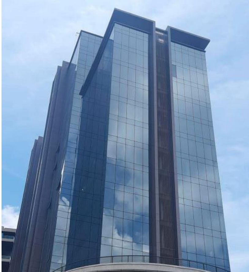
Tower 2 – OC received on 6 th Oct 2020; tenants started moving in during May 2021
