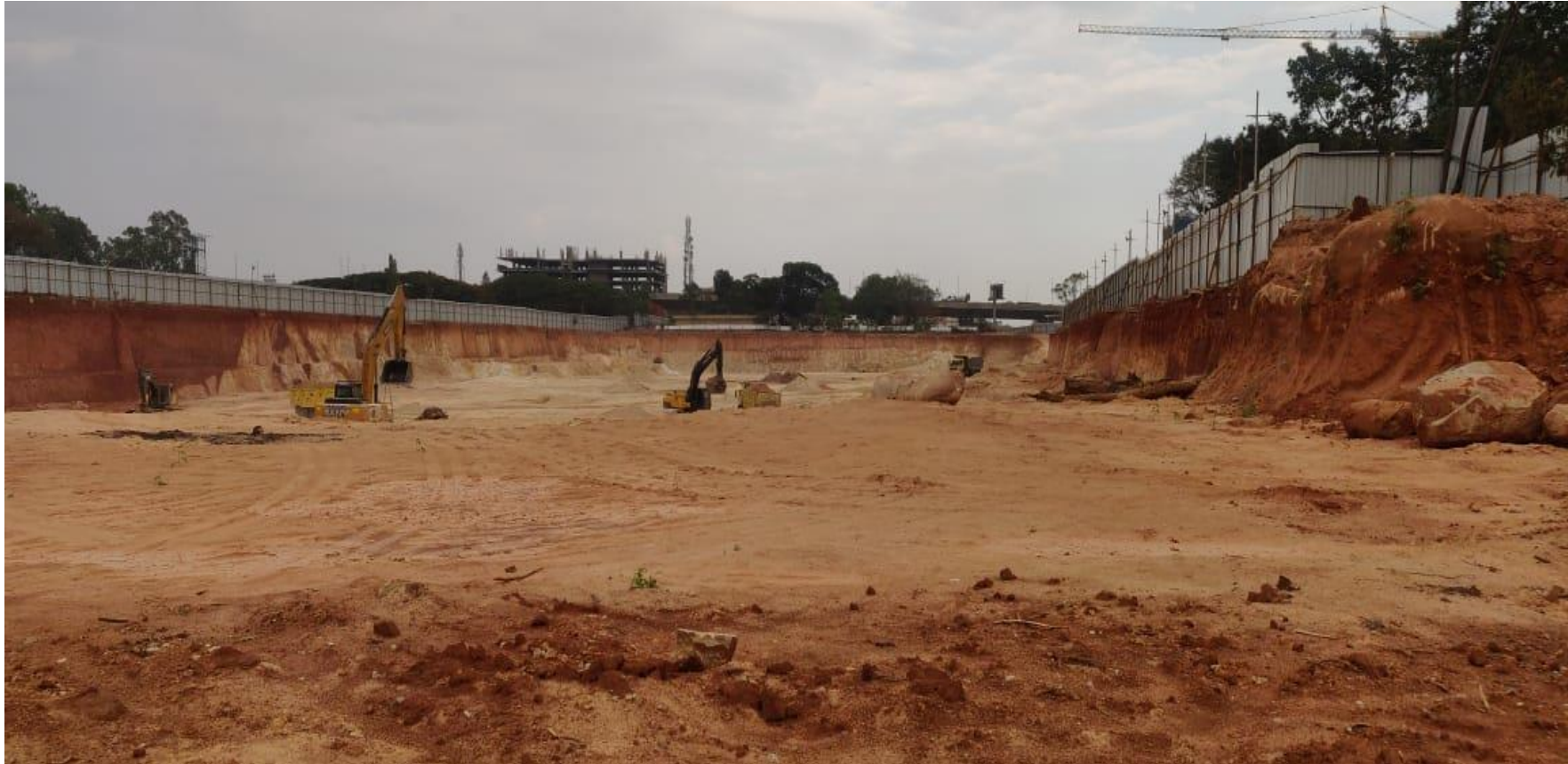
Excavation in progress
