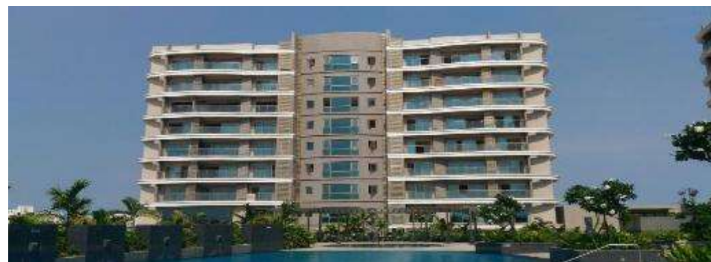
CREST TOWER A
