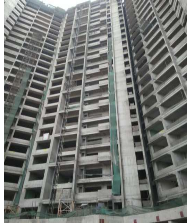
STRUCTURE WORK OF KESSAKU
