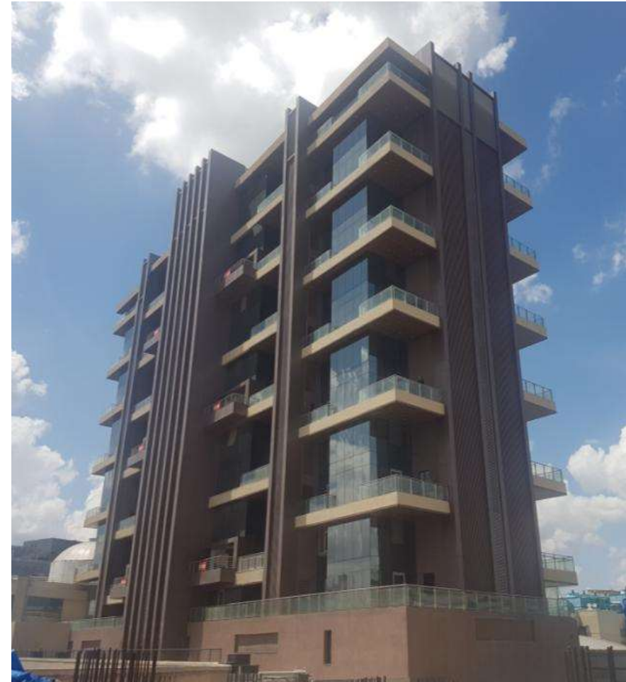
Fountainhead Tower 1 - Side
