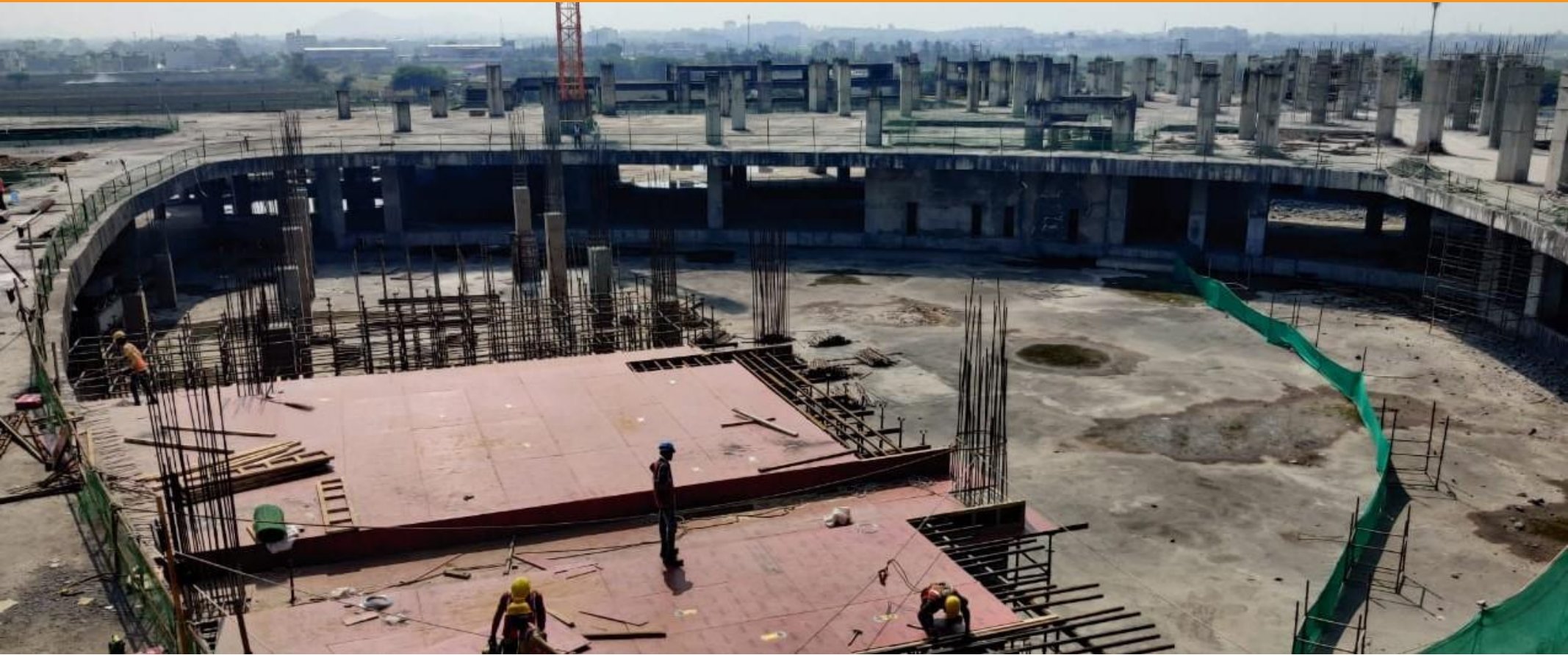
Construction in Progress
