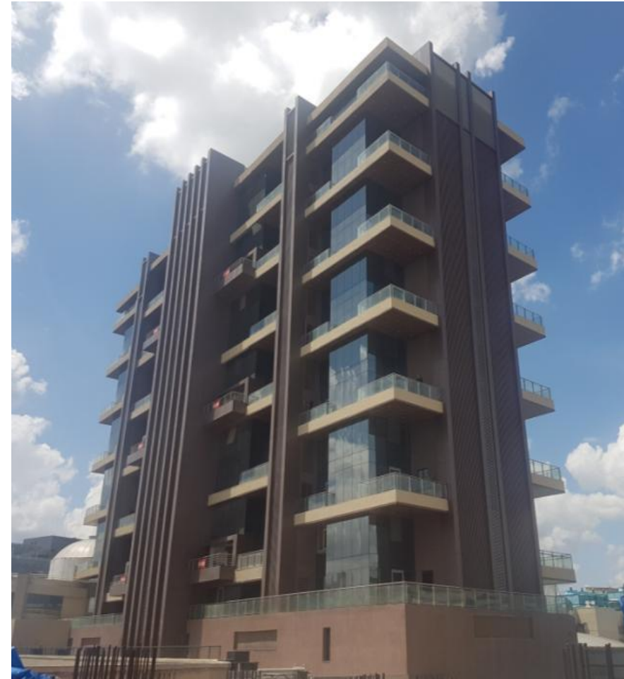
Fountainhead Tower 1 - Side
