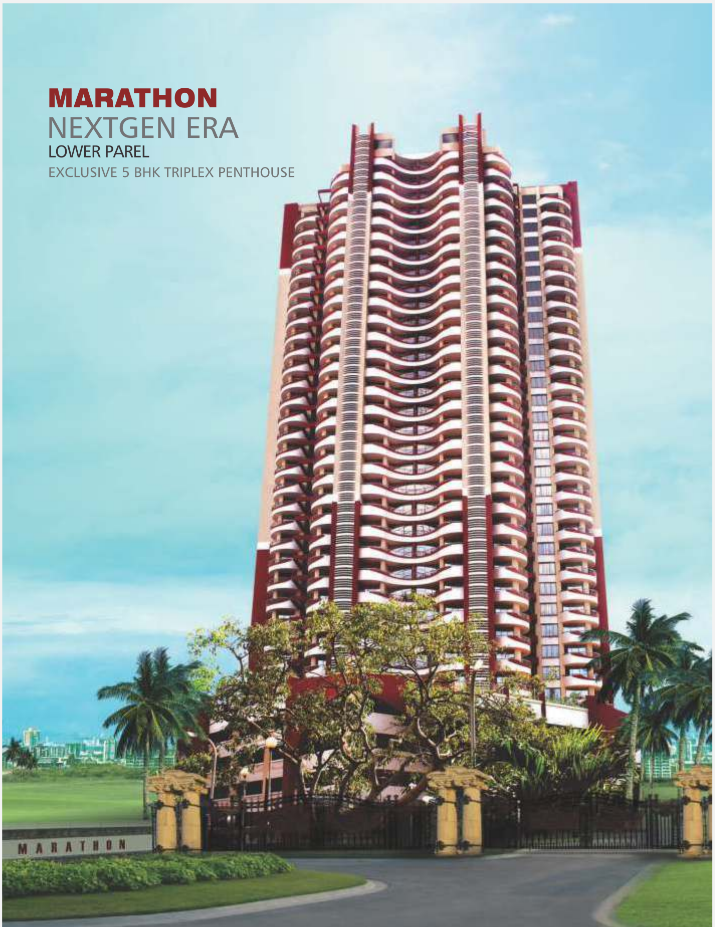
Actual Photograph - Elevation
