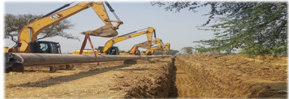
Setting up slurry pipeline
