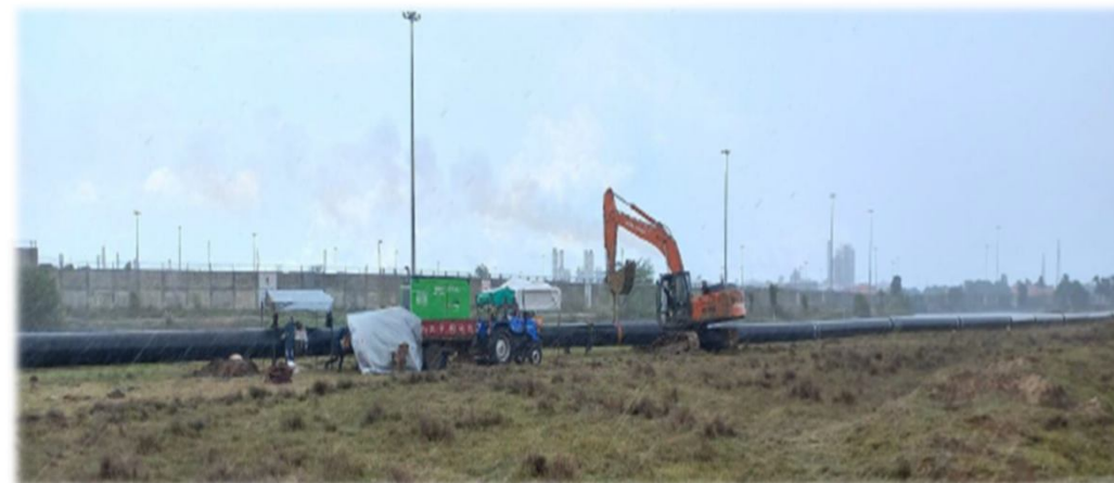
Setting up slurry pipeline
