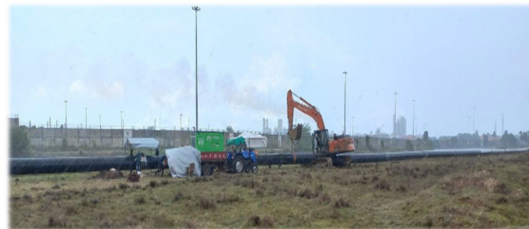
Setting up slurry pipeline
