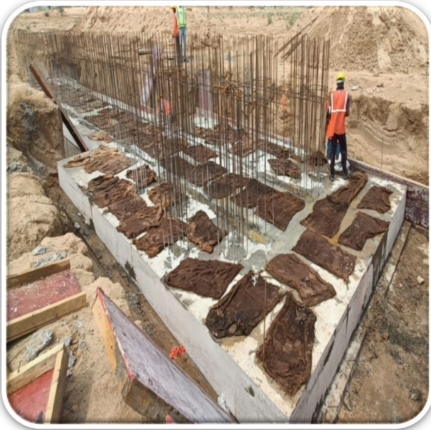
Power Transformer Foundation
