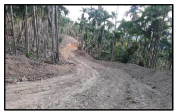
CONSTRUCTION OF ROAD
