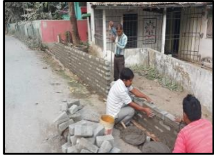
BOUNDARY WALL CONSTRUCTION
