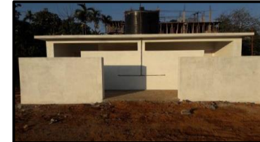
PUBLIC TOILET BLOCK
