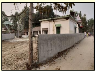
BOUNDARY WALL CONSTRUCTION
