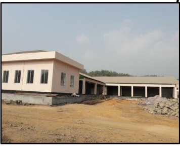
CONSTRUCTION OF MARKET
