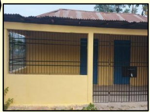
SCHOOL BUILDING RENOVATION
