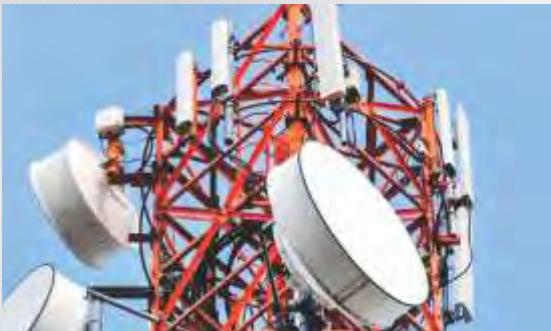
Project Details: Telecom Tower Erection Product Used: Steel Tubes
