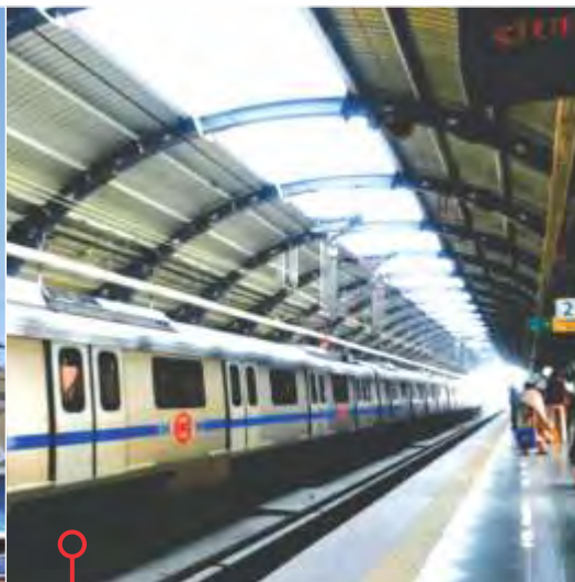
Station Structure & Railing- Delhi Metro
