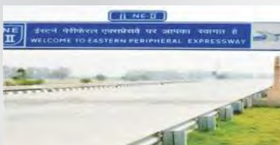
Project Details: Highway Crash Barriers along the long stretch of Eastern Peripheral Expressway, Uttar Pradesh Product Used: Highway Crash Barrier
