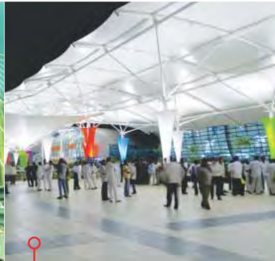
Tensile Membrane Structures- Mumbai Airport
