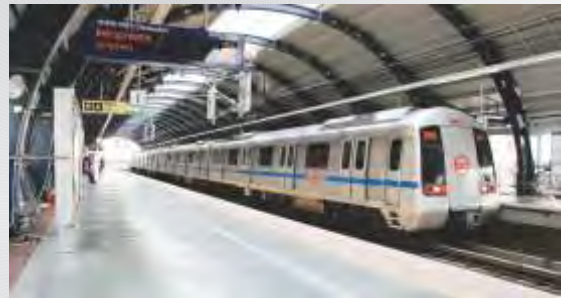
Project Details: Metro Station structure at Delhi Metro's Phase III Product Used: Hollow Sections
