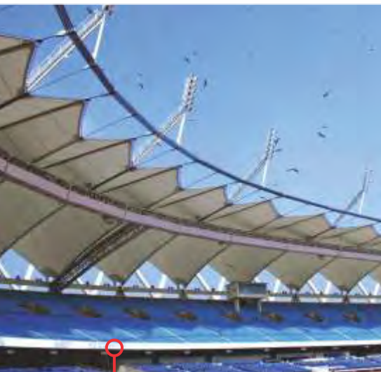
Main Supporting Structures- Common Wealth Stadium
