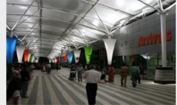
Tensile Membrane Structures- Mumbai Airport
