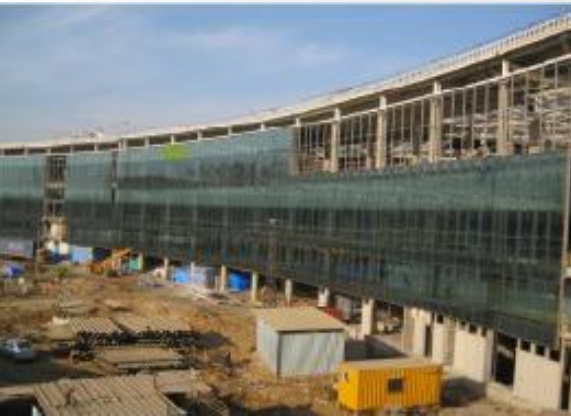
Curtain Walling Structure- Mumbai New Airport Terminal
