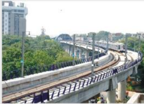
Station Structure & Railing- Delhi Metro
