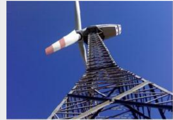
Towers- Suzlon Wind Farms
