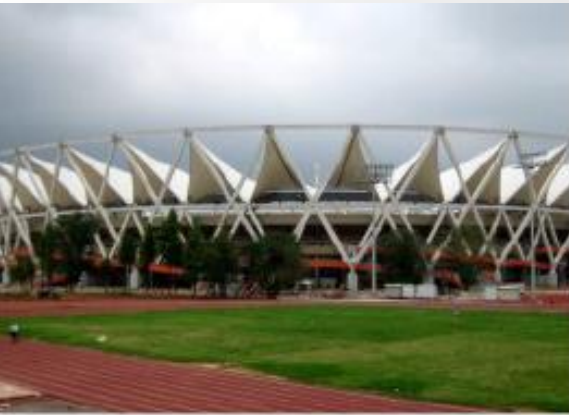
Main Supporting Structures- Common Wealth Stadium
