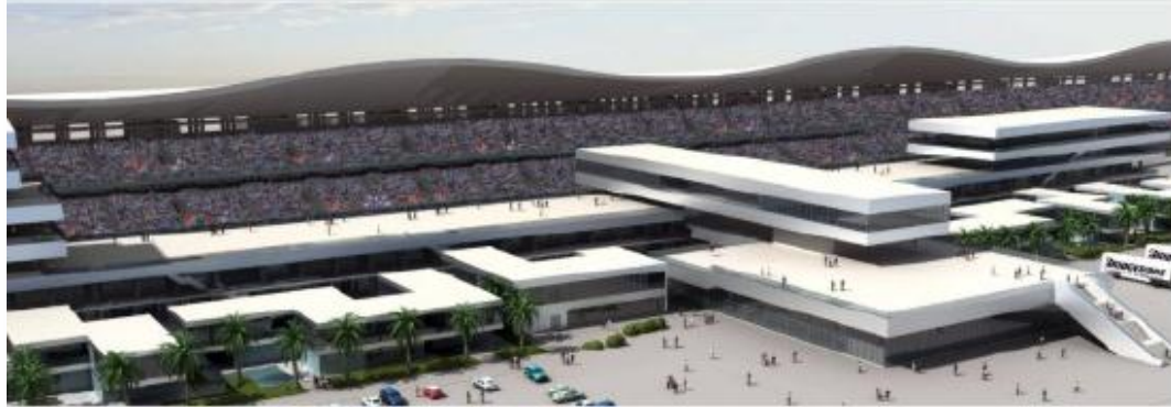
Grandstand Roofing Structure- Buddh International Circuit
