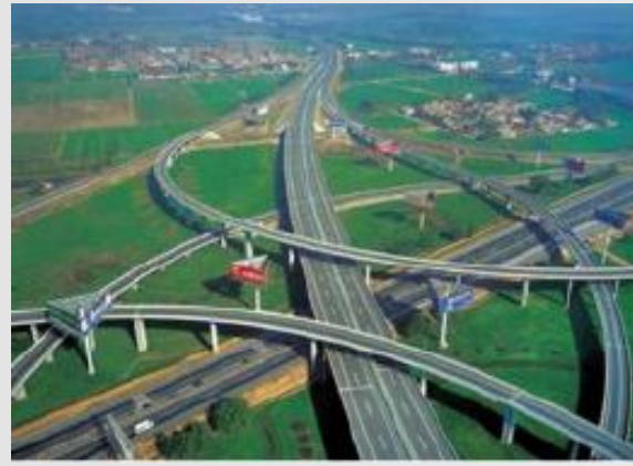
Crash Barriers- Yamuna Expressway
