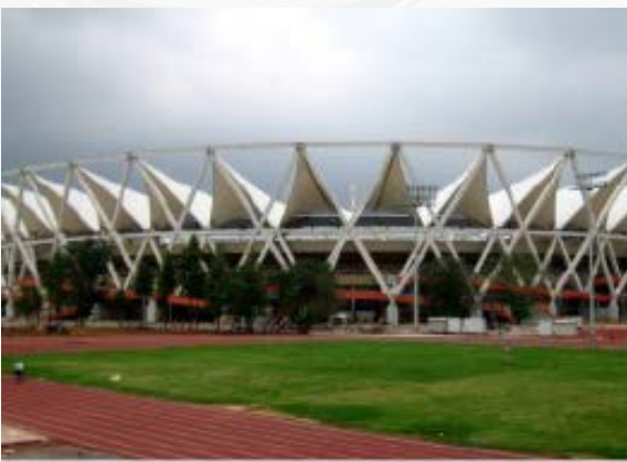
Main Supporting Structures- Common Wealth Stadium
