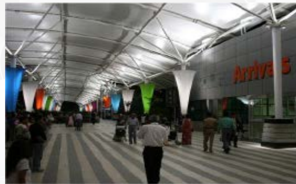
Tensile Membrane Structures- Mumbai Airport
