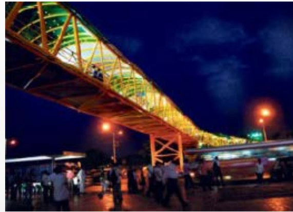
Walkways – Mumbai Skywalks
