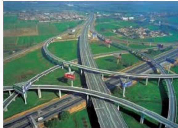
Crash Barriers- Yamuna Expressway
