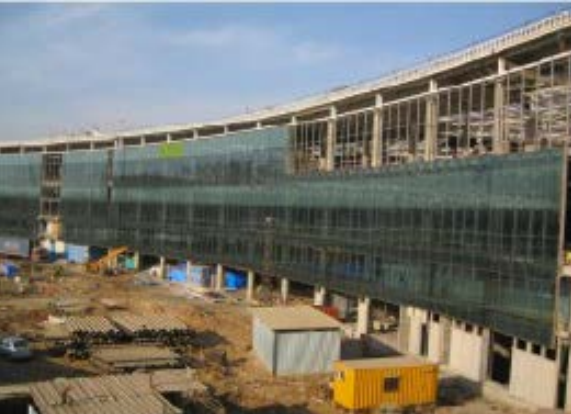
Curtain Walling Structure- Mumbai New Airport Terminal
