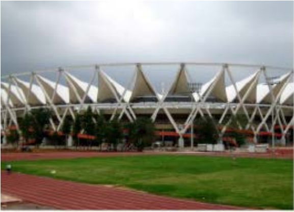
Main Supporting Structures- Common Wealth Stadium
