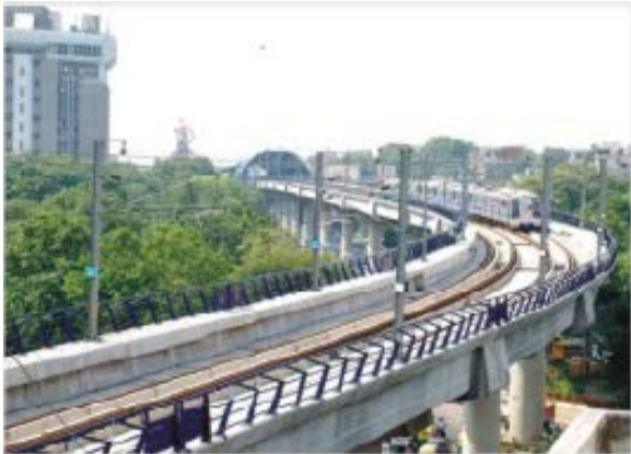
Station Structure & Railing- Delhi Metro
