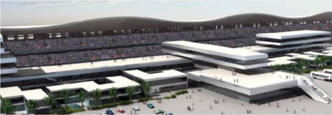
Grandstand Roofing Structure- Buddh International Circuit
