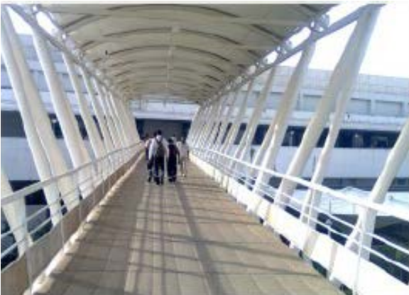
Structural Support Members- Foot Over Bridges in Delhi
