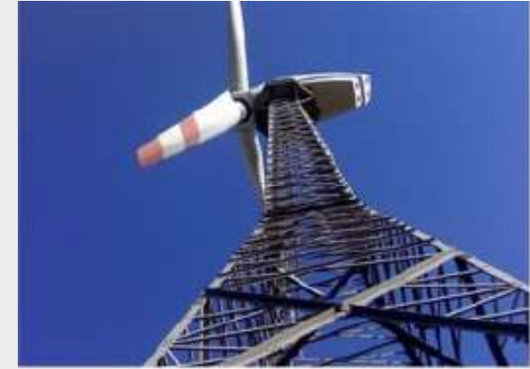
Towers- Suzlon Wind Farms
