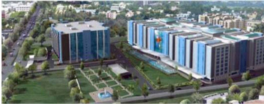
Fire Fighting Pipes- Seven Hills Hospital Mumbai
