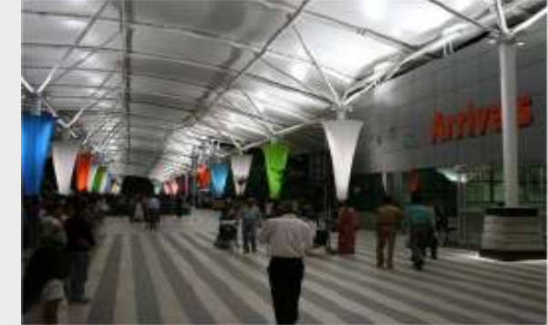
Tensile Membrane Structures- Mumbai Airport
