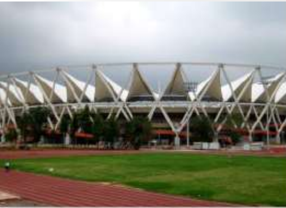
Main Supporting Structures- Common Wealth Stadium
