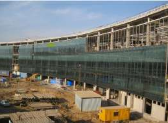
Curtain Walling Structure- Mumbai New Airport Terminal
