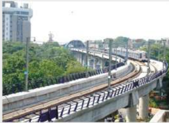
Station Structure & Railing- Delhi Metro
