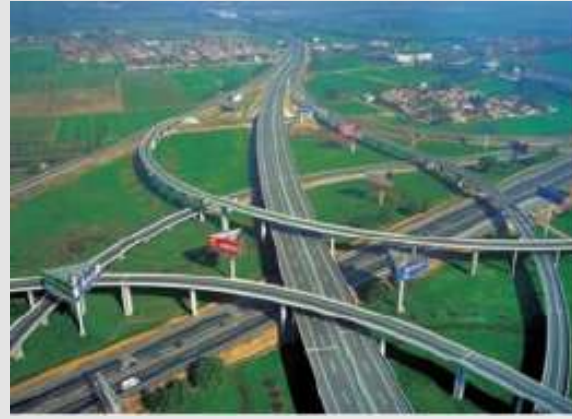
Crash Barriers- Yamuna Expressway
