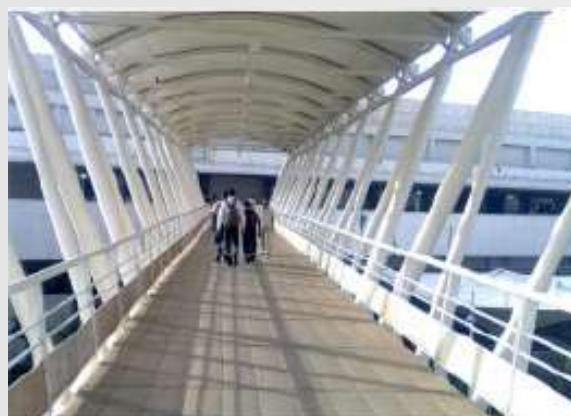
Structural Support Members- Foot Over Bridges in Delhi
