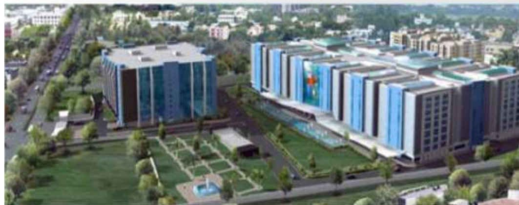
Fire Fighting Pipes- Seven Hills Hospital Mumbai
