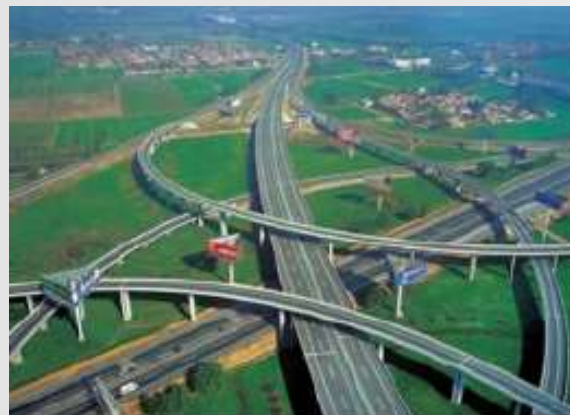
Crash Barriers- Yamuna Expressway
