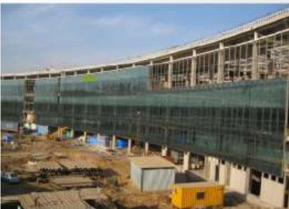
Curtain Walling Structure- Mumbai New Airport Terminal
