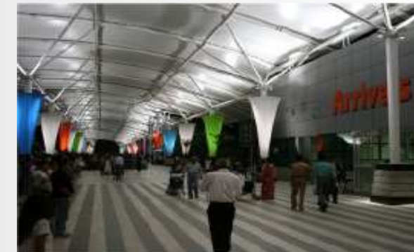
Tensile Membrane Structures- Mumbai Airport
