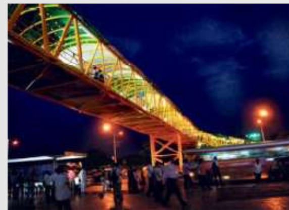
Walkways – Mumbai Skywalks
