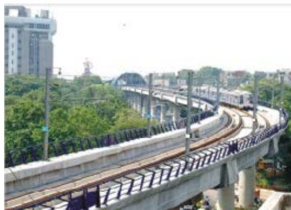
Station Structure & Railing- Delhi Metro
