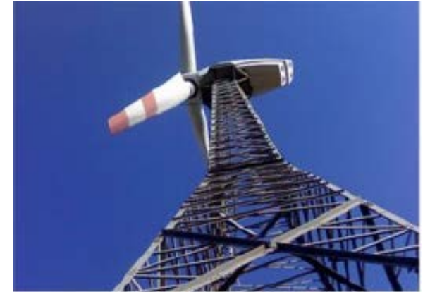
Towers- Suzlon Wind Farms
