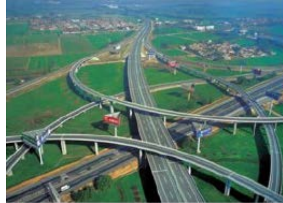
Crash Barriers- Yamuna Expressway
