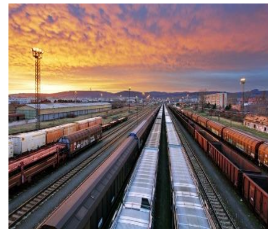
Dedicated Freight Corridor
