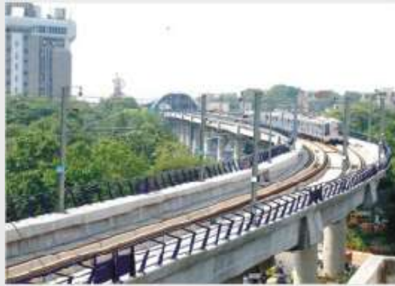
Station Structure & Railing- Delhi Metro
