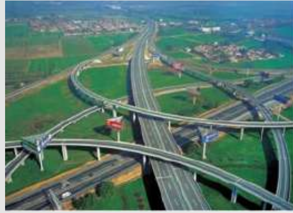
Crash Barriers- Yamuna Expressway
