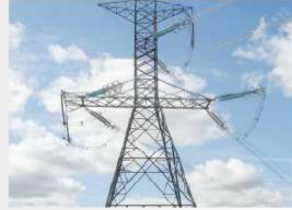
Substation Tubular Structure- Powergrid Corporation Ltd.
