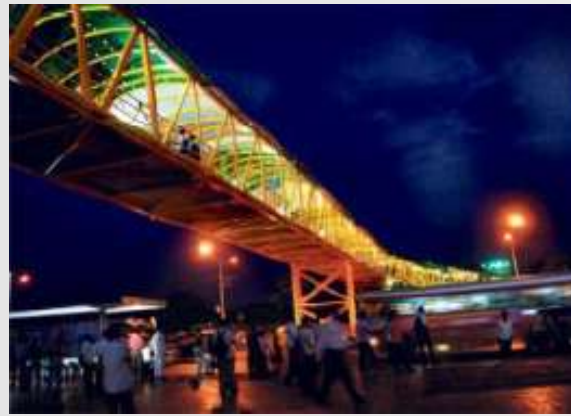
Walkways – Mumbai Skywalks
