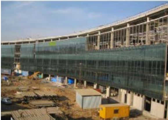
Curtain Walling Structure- Mumbai New Airport Terminal
