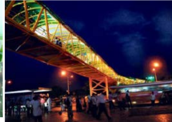
Walkways – Mumbai Skywalks
