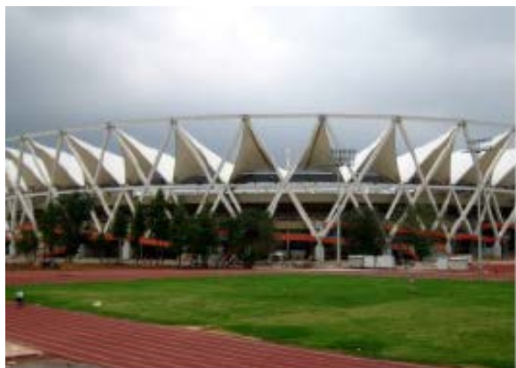
Main Supporting Structures- Common Wealth Stadium
