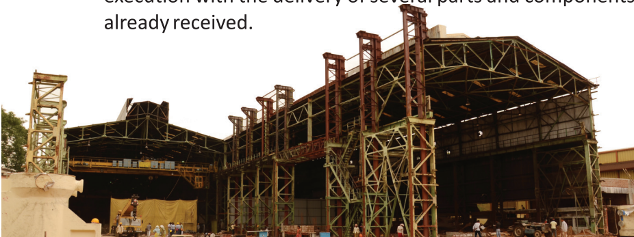
Construction activities in full swing for erection of 6000 T Forge Press
