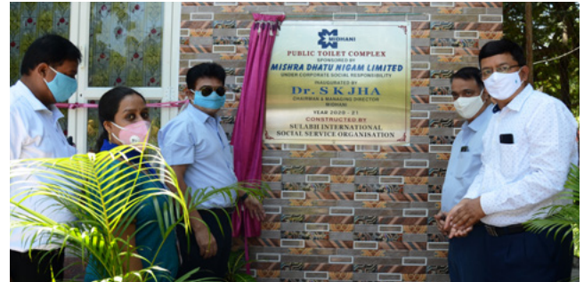
In line with Swachh Bharat Mission, Dr. S.K. Jha, Chairman & Managing Director, MIDHANI inaugurating Public Toilet Complex (for Gents & Ladies) constructed under Corporate Social Responsibility
