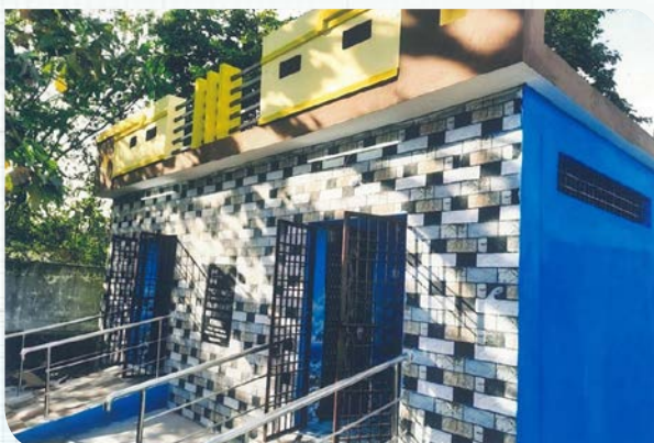
◀ Construction of toilet at ZPSS Narsapuram, Kothagudem District
