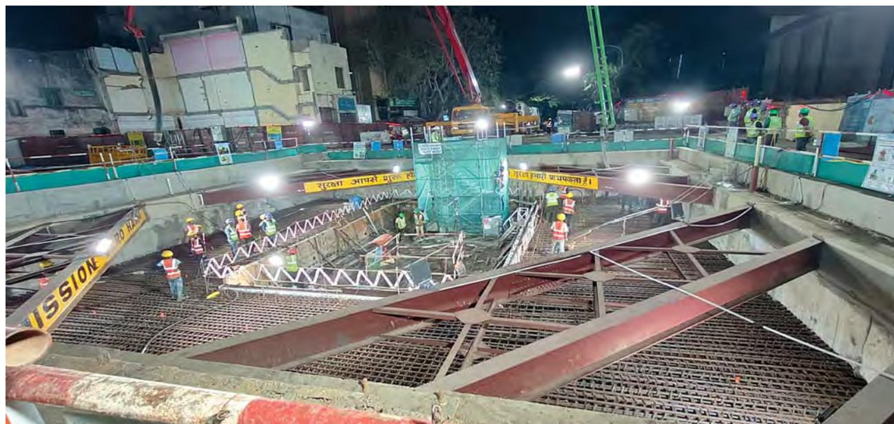
UG-04 – RK SALAI STATION (North shaft Roof slab casting in progress)
