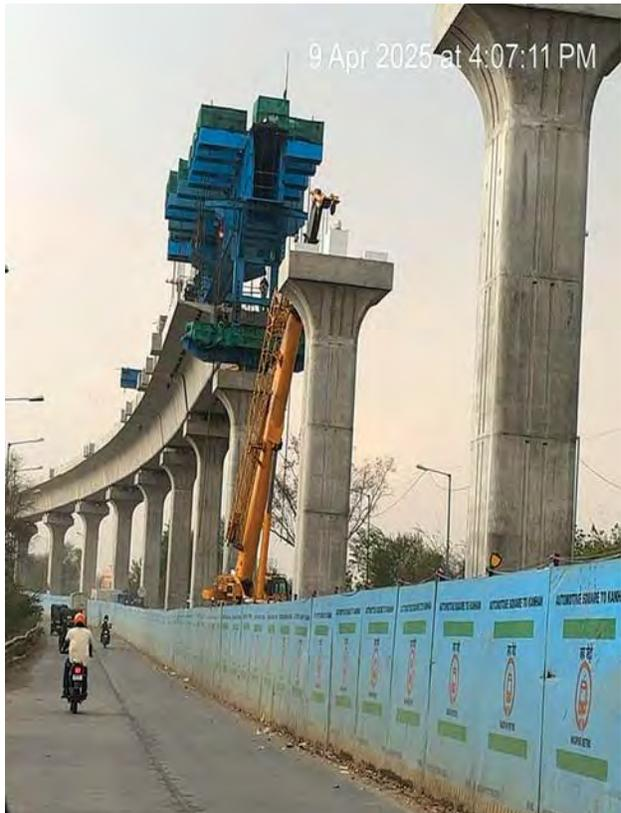
Work is going on in full swing in all packages. Major package pertains to construction of 6.92 km Viaduct (Only Civil Portion). It involves 238 number of spans. Around 45% of this package is complete. Launching of 56 spans (total 1.75 km) with 3 no's of LGs has been completed till date.
