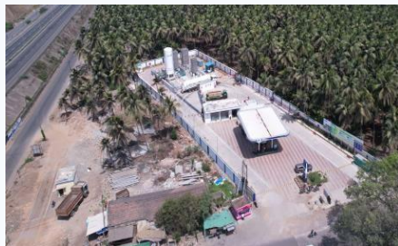
LNG/LCNG fuel stations
