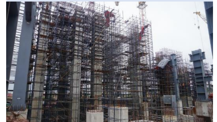
Unit #2 Turbine Generator Deck Column Casting
