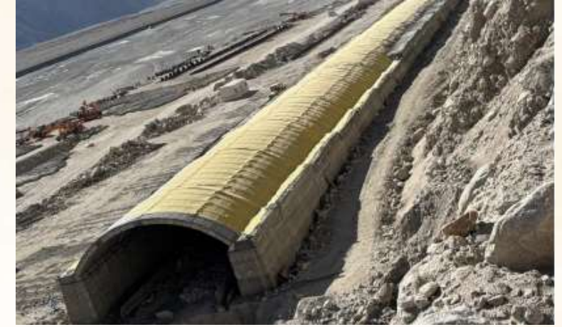
Leh, Ladakh - India's Longest Precast Cut- and-Cover Tunnel
