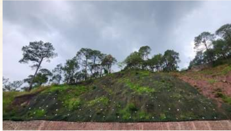
Slope Protection Work at Parwanoo - Solan section of NH 5, Himachal Pradesh
