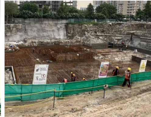
Tower 4 - As on 24 th July 2025 - The piling work has been completed, and raft foundation work is in progress.
