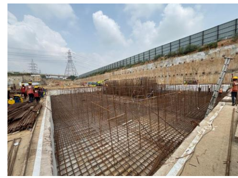
Tower 4 - As on 24 th July 2025 - The piling work has been completed, and raft foundation work is in progress.
