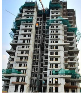
Tower 2 - As on 24 th July 2025 – Nineteenth floor slab is being casted.
