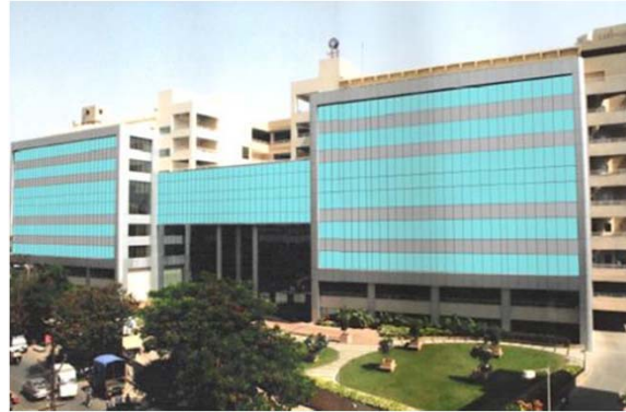
Karve Road, Pune (operational)
