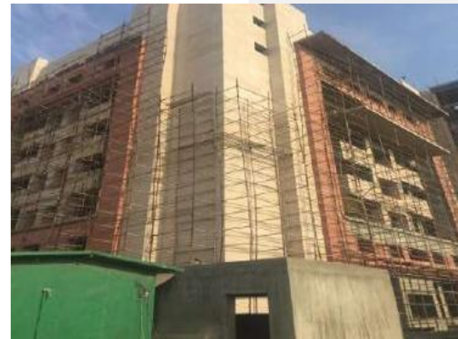
Finishing works of NHAI Dwarka
