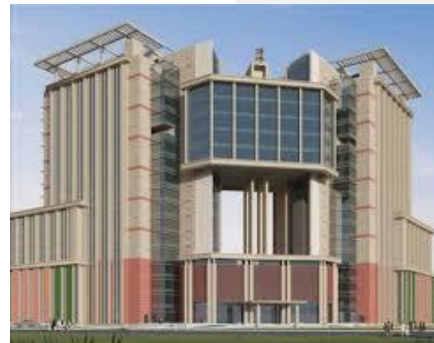
Construction of Delhi Police Headquarters
