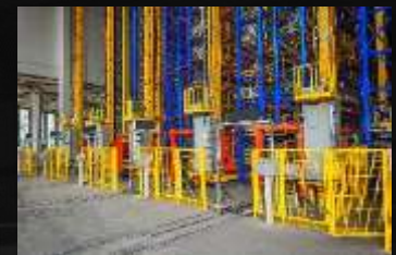
ASRS CRANE BASED
