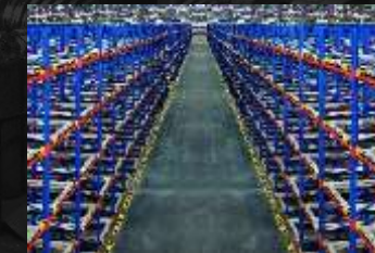
PUSH BACK PALLET RACKING
