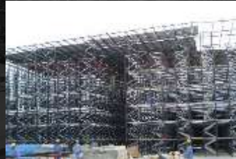
RACK SUPPORTED WAREHOUSES
