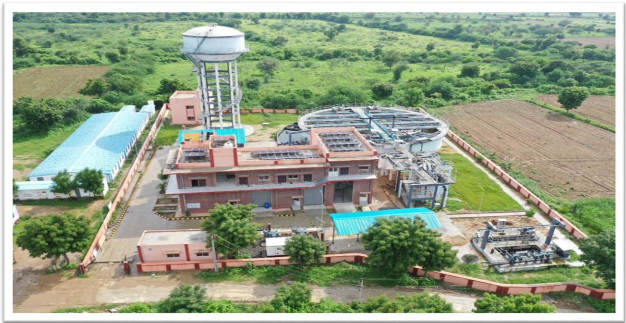
5 MLD STP Plant at Sirohi, Rajasthan
