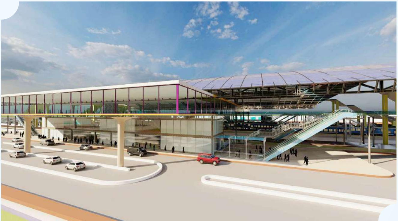
Faridabad Railway Station Project Under Way
