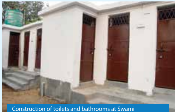
Construction of toilets and bathrooms at Swami Shahjanand Trust, India
