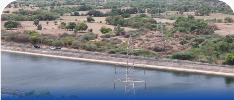
220 kV River Crossing Project (Government)
