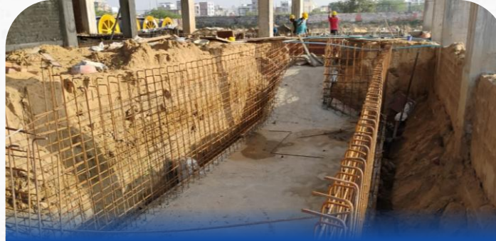
132 kV GIS at Pratapnagar, Jaipur
