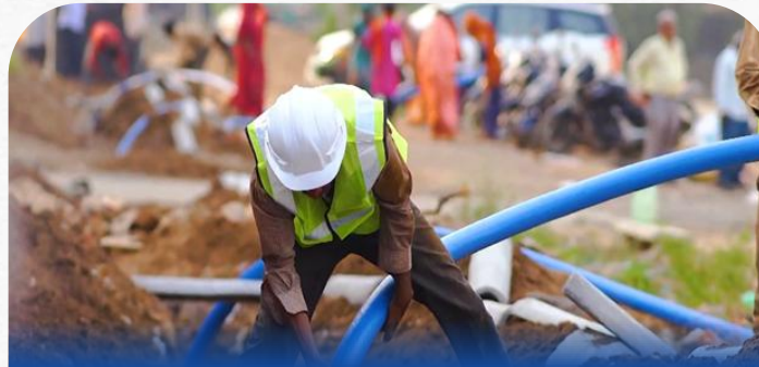
Underground cable laying for Robust network for DGVCL
