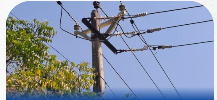
Conversion of overhead 11 kV conductor to MVCC
