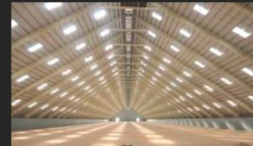
Approx 90,000 sq. m. 'A' frame structure with a centre height of 42 metres and clean span of 84 metres specially designed for the sugar storage requirements for a major Indian sugar company in Kandla, Gujarat
