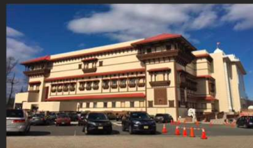
Over 18,000 sq. m. PEB installation for a temple at New Jersey, US
