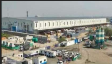
Over 57,000 sq. m. PEB installation for a warehouse, for a multinational e-commerce company at Ahmedabad, Gujarat
