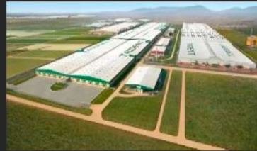
Over 285,000 sq. m. PEB installation for a textile plant for a major textile company at Hoshangabad, Madhya Pradesh
