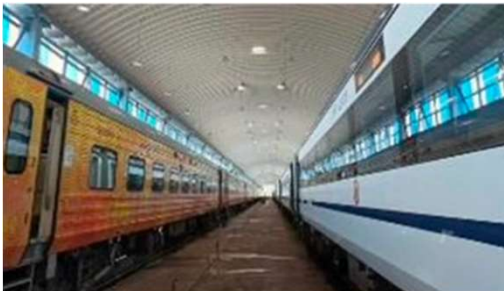
Vande Bharat Mumbai Central Pit Line Shed
