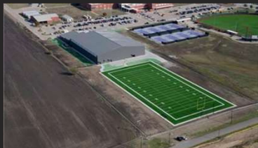
Over 5,500 sq. m. PEB installation for an indoor multi-use facility at Texas, US
