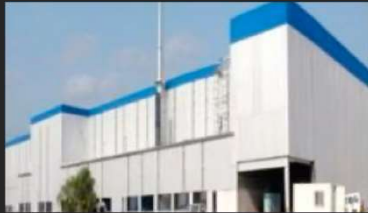
Over 62,000 sq. m. PEB installation for the automobile manufacturing plant of a global automobile manufacturer located at Ahmedabad, Gujarat
