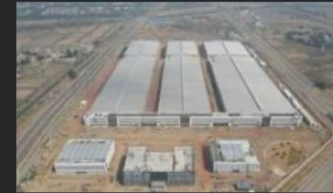
Over 125,000 sq. m. PEB installation for a multinational home appliance manufacturer based out of Noida
