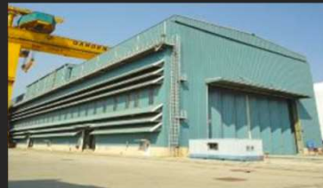
Approx 3,000 sq. m. PEB installation with a retractable (openable) roof structure for a Kolkata based shipyard
