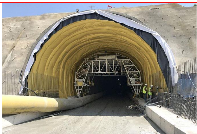
Waterproofing services of tunnel at Maharashtra
