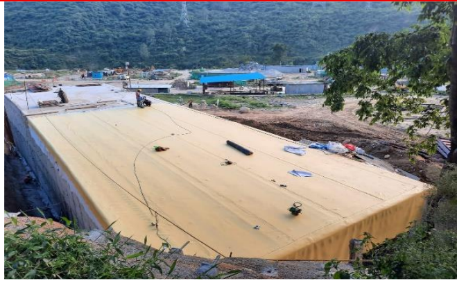
Waterproofing services of rooftop at Arunachal Pradesh
