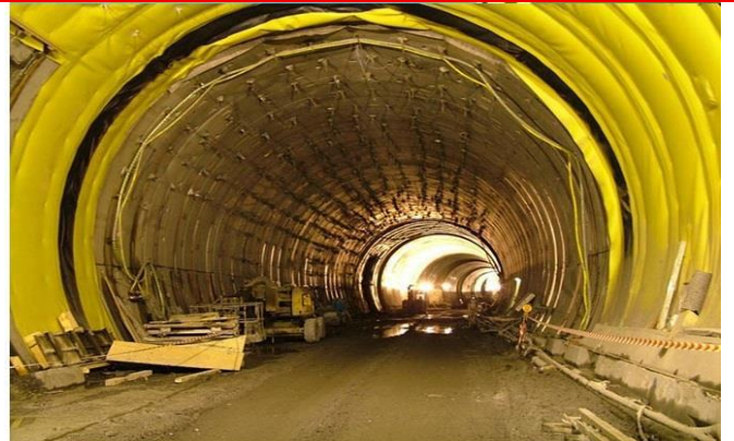
Waterproofing services of tunnel at Odisha
