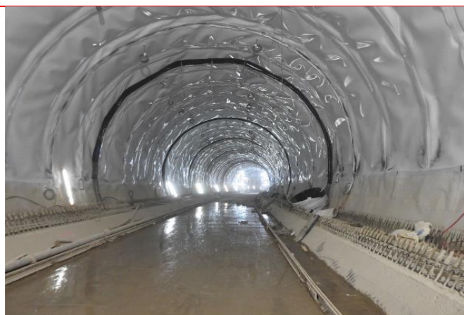
Waterproofing services of tunnel at Himachal Pradesh
