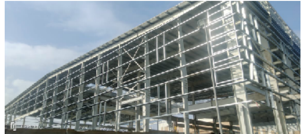
Khatalwada plant expansion building
