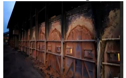
Battery with 32 Ovens
